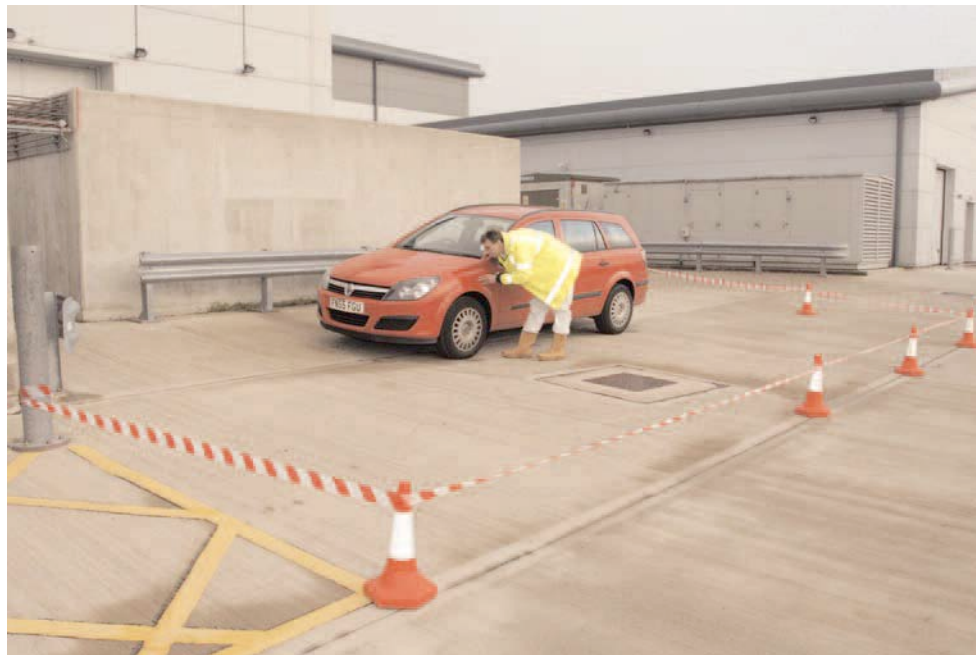
Figure 1 Well-defined external area ready for SMART spraying
